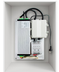
Control Box & Power Supply housed in cabinet
